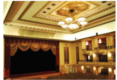
The Grand Ballroom was the largest space of its kind in 1931. When combined with the adjoining foyers, the 35,000 square-foot-space can easily accommodate over 6,000 guests. The two tiers of private boxes feature Art Deco interpretations of classical bas-reliefs. Other ornamentation in the space includes typical Art Deco motifs: leaping gazelles, frozen fountains, and stylized foliage.
