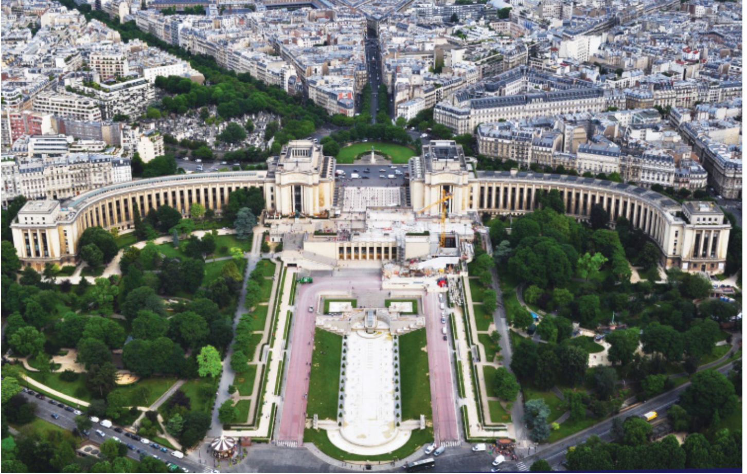
Aerial view of the Palais de Chaillot, Léon Azema, Jacques Carlu, and Louis-Hippolyte Boileau, architects, 1937. All Photos: Meghan Weatherby
