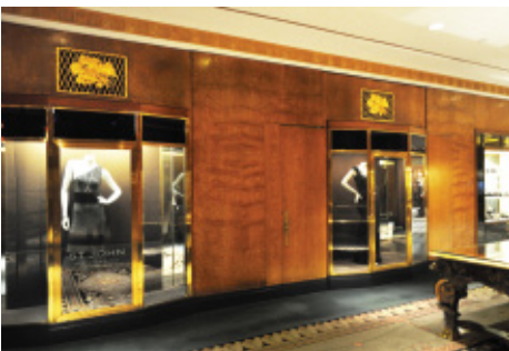
Concealed shelving and compartments, as well as adaptable storage, were typical of American Art Deco residential spaces. As seen in the East Corridor, the doors have been disguised by the same wood paneling as the walls.
