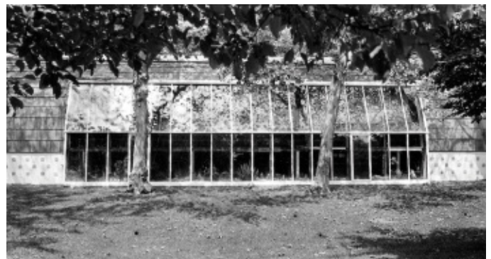
The house designed for Robert Motherwell by Pierre Chareau. Courtesy of Barney Rosset Estate. The East Hampton, Long Island home combined a surplus World War II Quonset hut with a window from an industrial greenhouse, concrete blocks, and plywood.
