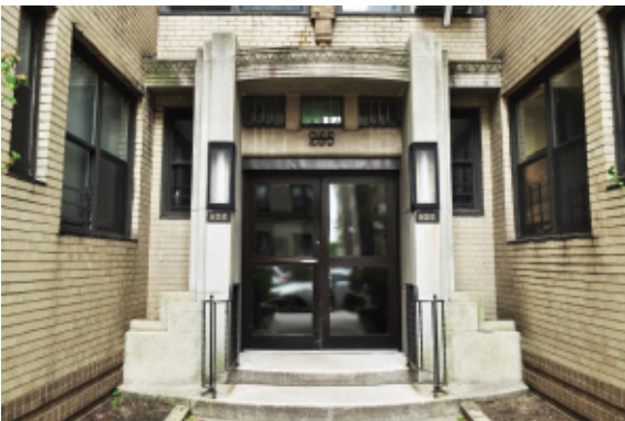
14. 265 Cabrini Boulevard The typical Art Moderne entrance of this 1936 apartment building by Miller & Goldhammer combines curved horizontal bands and straightedged verticals with overlapping rectangles near the bottom and alternating triangles across the top. The original doors, unfortunately, have disappeared.
