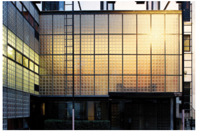
Pierre Chareau and Bernard Bijvoet, Maison de Verre, 1928-1932. The residence, designed for the Dalsace family, is sheathed in translucent textured glass brick. Photo: © Mark Lyon
