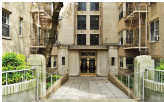
19. Fort Tryon Gardens, 720-730 Fort Washington Avenue These two apartment buildings from 1938-39 were also designed by Jacob M. Felson. They typify end-of-the-decade Art Deco by forgoing bright colors and vertical lines and focusing instead on simple white brick, concave curves and sunken, central entrances. The lobby sports a mural inspired by the neighborhood's Revolutionary War history.
